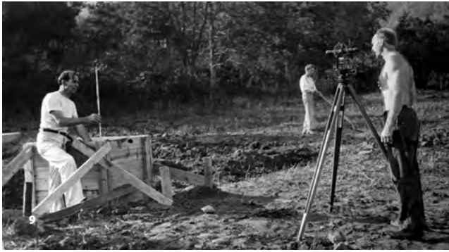
9 Lawrence Kocher y Ted Dreier replanteando el Studies Building de Kocher, c. 1940. / Lawrence and Ted Dreier doing revisions on Kocher's Studies Building , c. 1940. Fuente / Source: Western Regional Archives, State Archives of North Carolina (WRA/SANC).
